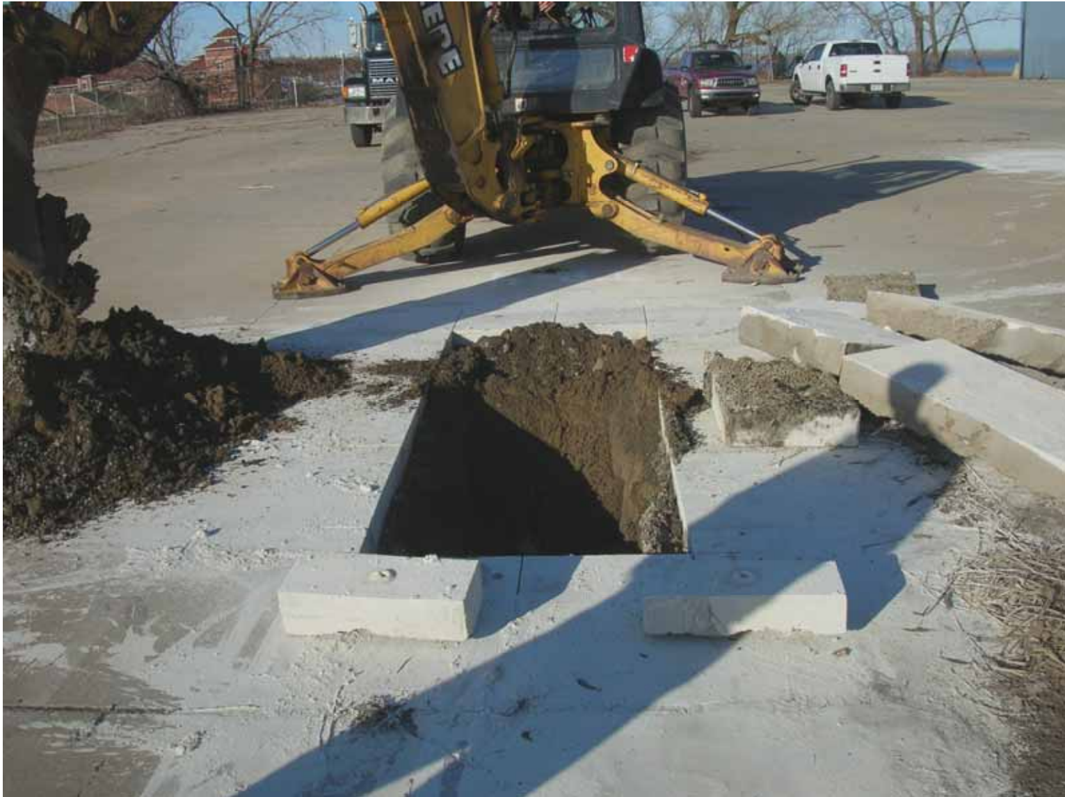
Test Pit TP-4
