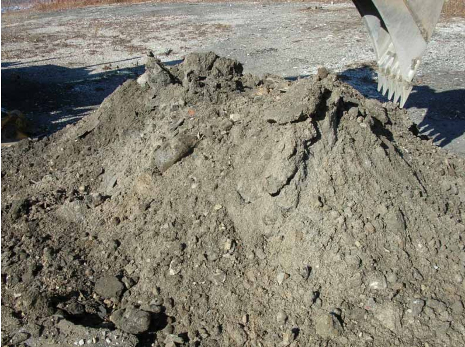
Test Pit TP-2 Waste Pile
