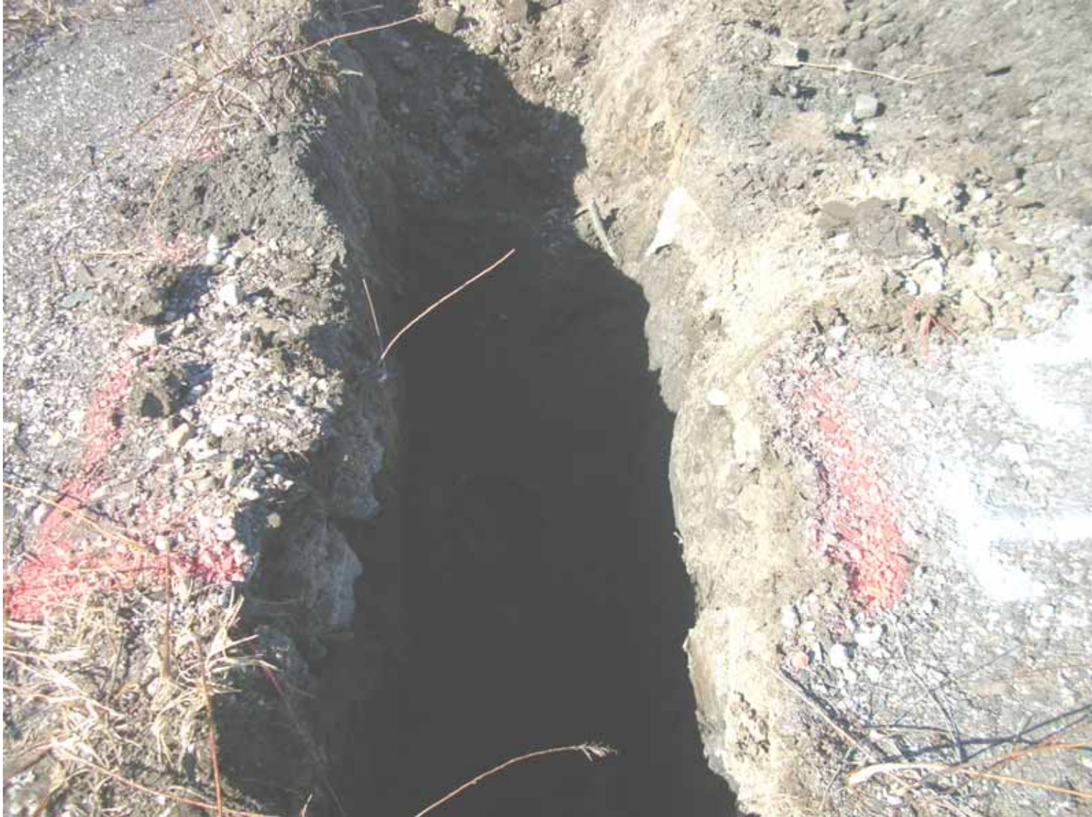
Test Pit TP-1
