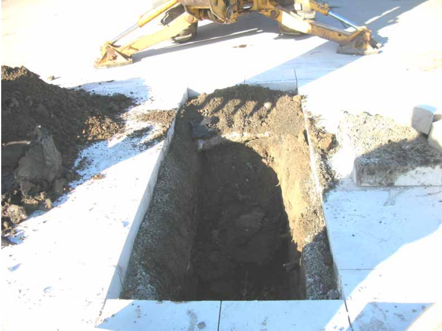
Test Pit TP-3
